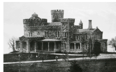
A. A. Turner, Herrick residence, Villas on the Hudson, 1860
